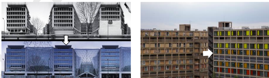
Figure 4.18 Example of before and after of refurbishment projects at 55 Baker Street (left) and Park Hill (right).
